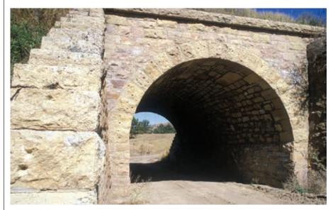
Grade-separated crossings include both underpasses and overpasses to allow pedestrians and cyclists to cross a highway without interfacing with motorists. To be successful, the crossing needs to provide direct access, have clear sight lines, include lighting for safety and address drainage.
